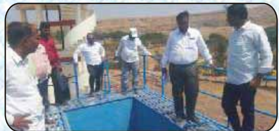
Social Audit under progress Field Visit at Water Treatment Plant at Village Hivare Block Purandar District Pune on 24/02/2020
